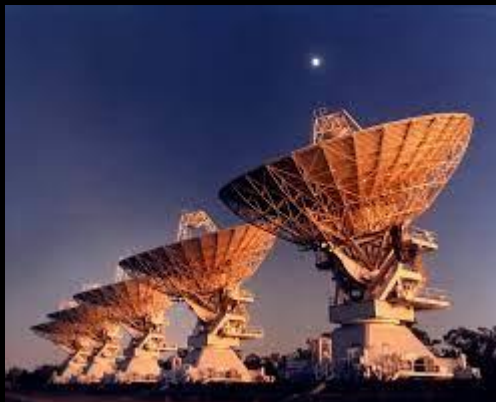
SKA Australia Telescope Facility
